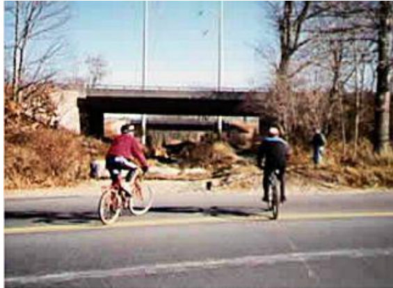
Location Of Phase 2 At 495 Overpass
